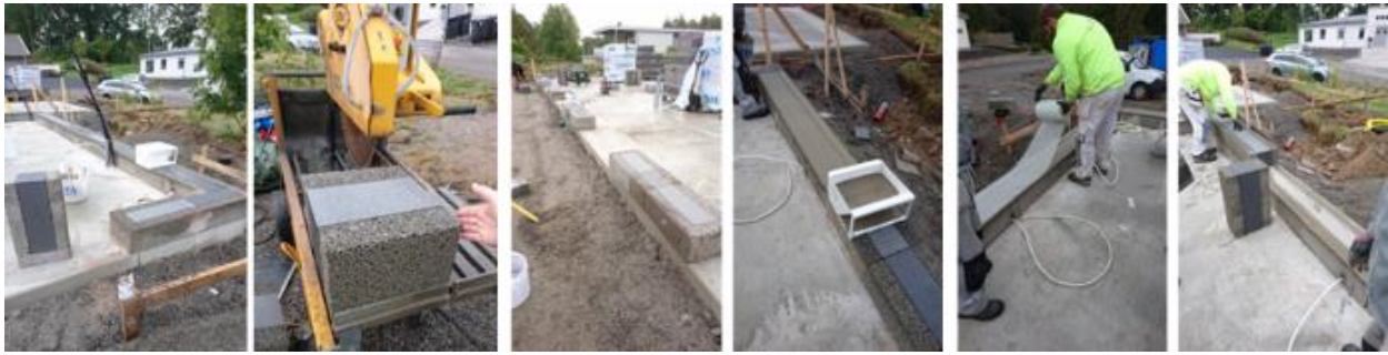
Figure 2. Steps in the manual masonry process in the Finja Exakt block system. From left to right: a) First layer. b) Customization of blocks. c) Door openings. d) Mortar application. e) Reinforcement application. f) Customization for cabling. [12]
