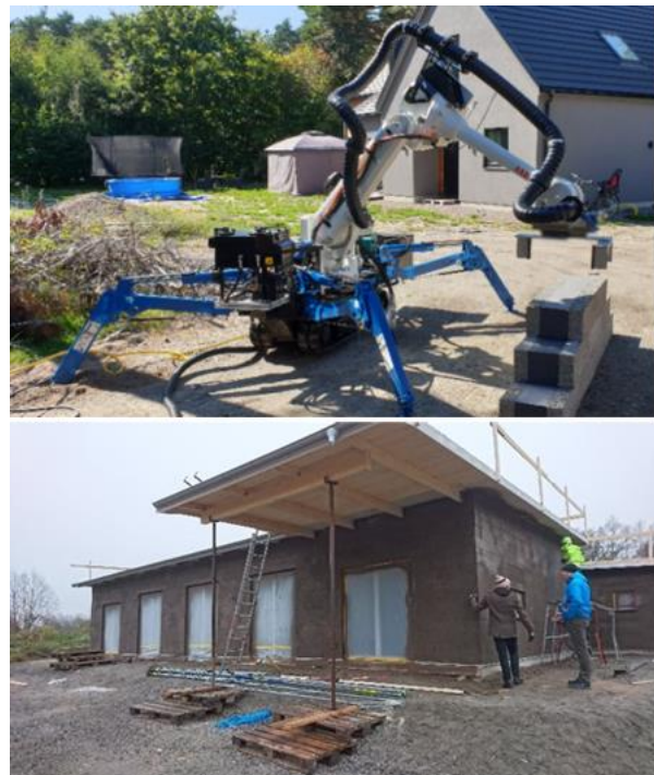
Figure 1. The mobile robot system Bettan (top) and the house type targeted by the robotized Finja Exakt build system (bottom) [11].
